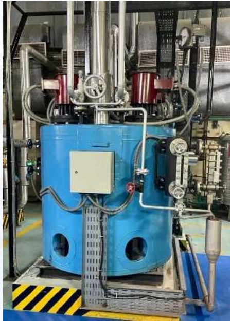
RE Operated Electrical Boiler (Fuel Switch, Zero Emissions)
